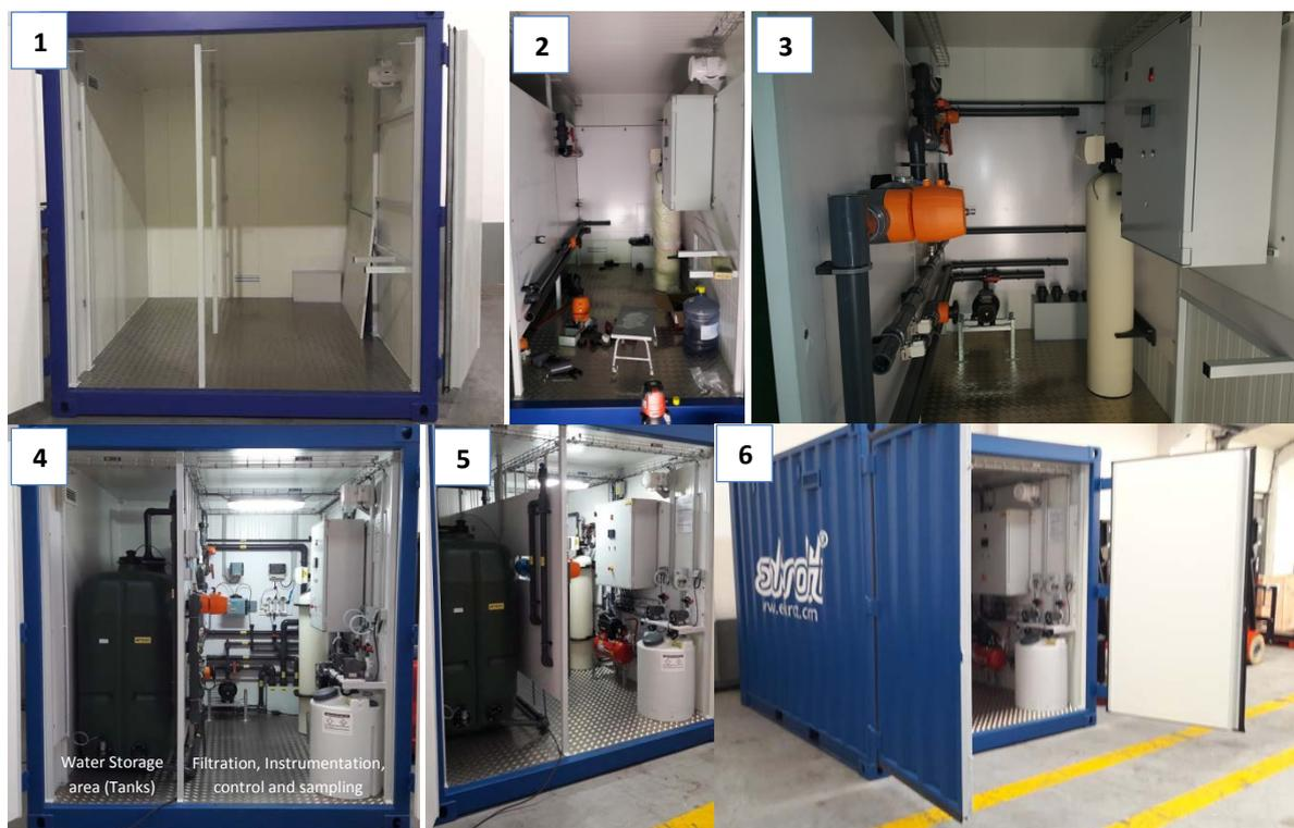
**Figure 2:** overview of the construction steps of the Treatment Stations that was engineered to Trancoso (TORRES) site
